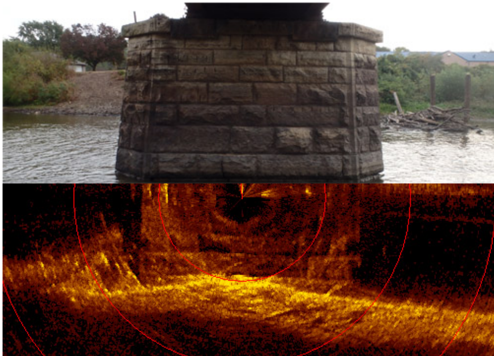
Photo 18 – Pier 25 – West face
