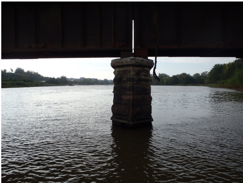
Photo 4 – Pier 22 – North face
