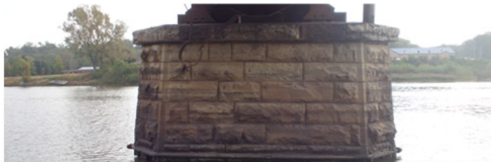
Photo 5 – Pier 22 – Upstream bullnose, facing East Note: Scour starting in front of the bullnose
