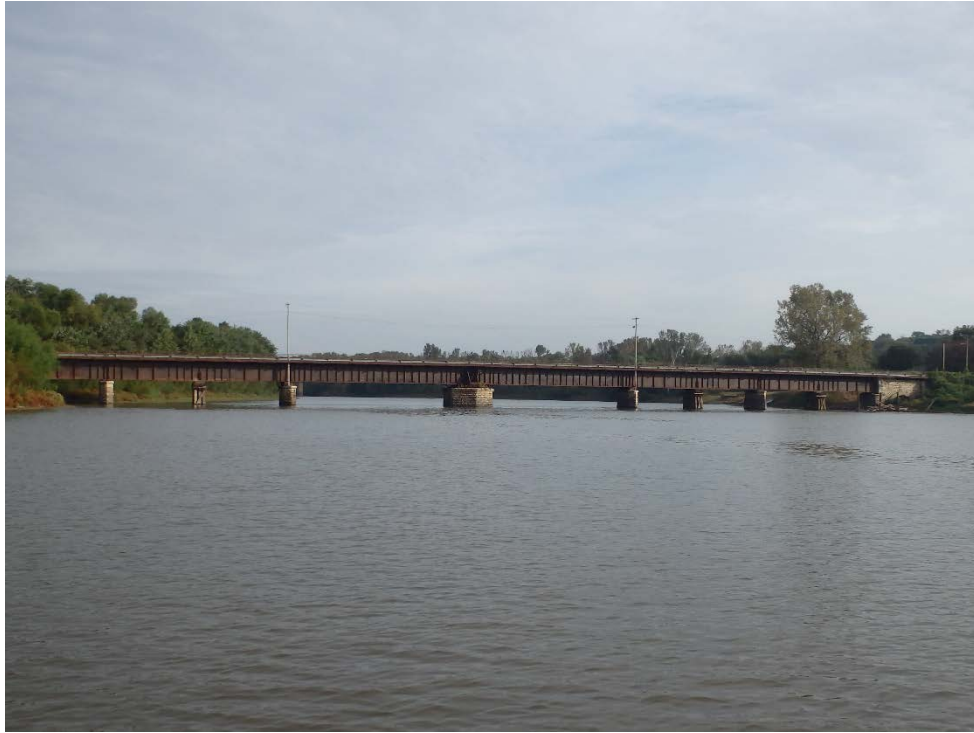
Photo 1 – Bridge profile – Downstream
