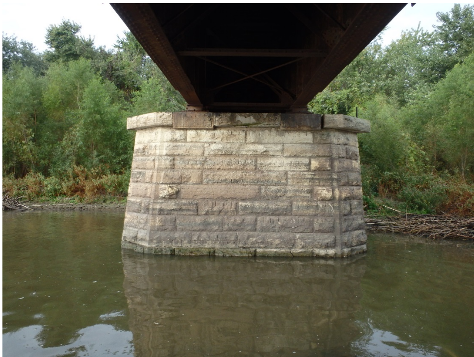
Photo 2 – Pier 21 – East face
