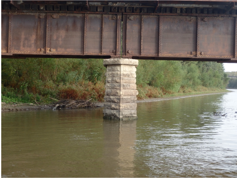
Photo 3 – Pier 21 – South face
